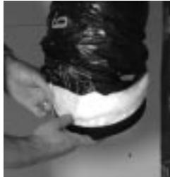
figure 7.3 Insert insulation inside the collar.
