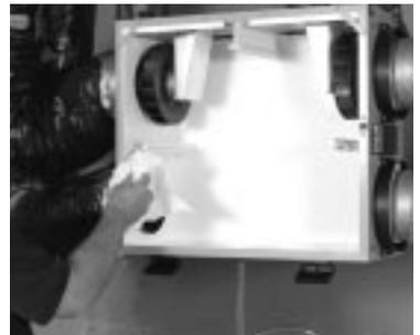
figure 17.4 Wash the Walls of the Unit
