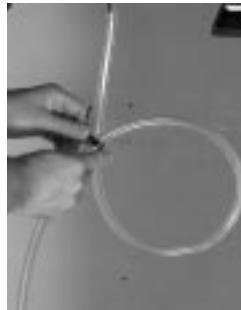
**figure 8.3** Make a loop in condensate line.
