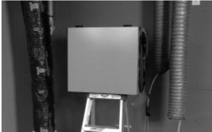
figure 5.1 Place HRV/ERV on a stepladder.
