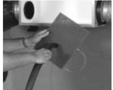
figure 17.2 Vacuum the Filters
