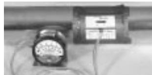
figure 13.5 Seal Air flow grid in duct with duct tape.
