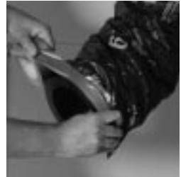
figure 7.4 Finish by taping the duct on the collar.
