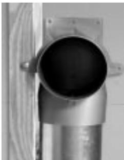
figure 11.2 Stack head elbow.
