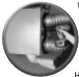
When using this application make sure that there is at least 6' between the fresh air and exhaust air connections of the HRV or ERV in the return air duct.
