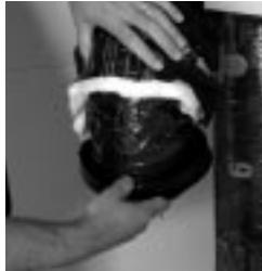
figure 7.2 Insert vinyl duct over the hooks and seal with a 30" tie wrap.
