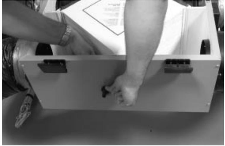
**figure 8.1** Hand screw the drain adapter
