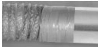
figure 6.2 Mount flex to rigid duct.
