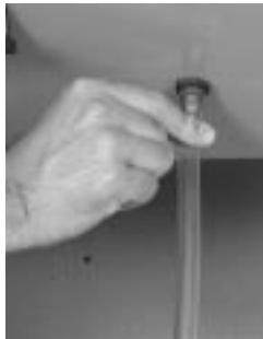
**figure 8.2** Insert condensate line.
