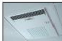
Drop ceiling installation
